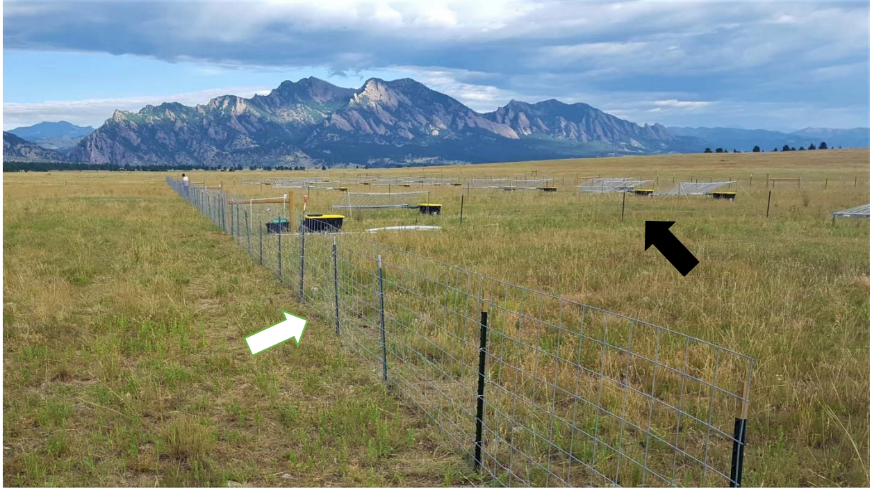
Fig. 2. Grazing blocks were constructed with permanent interior fences (barbed wire supported by H braces; black arrow) and removable exterior fences (cattle panels; white arrow).
