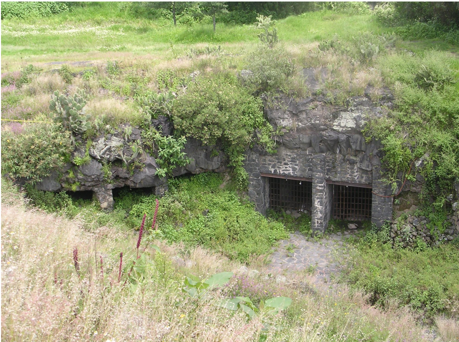
Figure 9 Cuicuilco building with lava flow.
