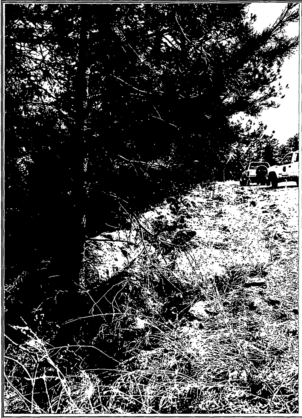
Fig. 12. A sediment dike lining a pull out on Flagstaff Road. The height of the dike, which was over 1 m, can be gauged by comparison with the tree in the foreground. This photograph was taken above GS 4.
