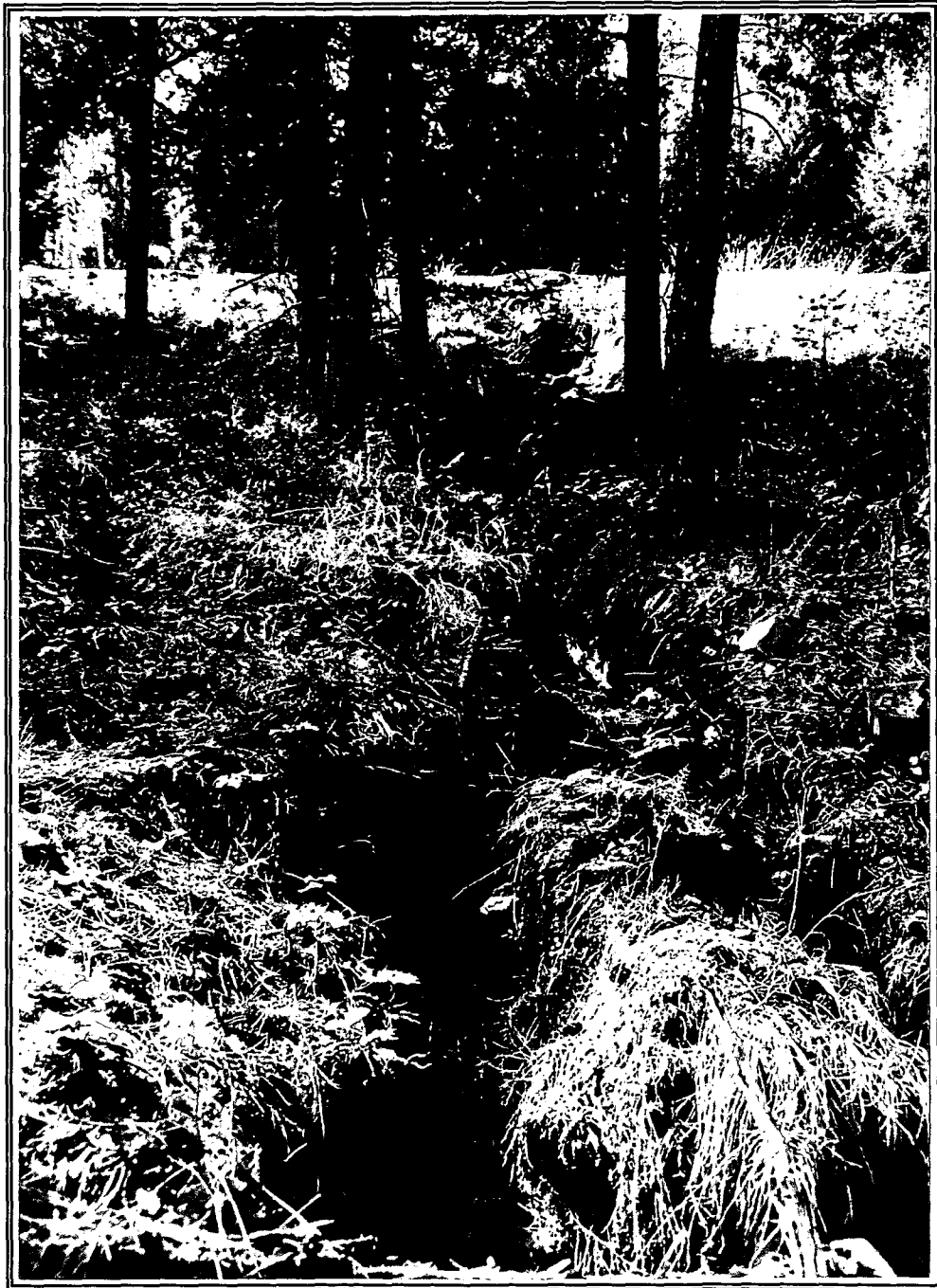
Fig. 11. Gully formation below the culvert feeding GS 4. The culvert opening can be seen just below the road grade, near the center of the photograph. This gully has formed in what was previously an undissected hill slope.
