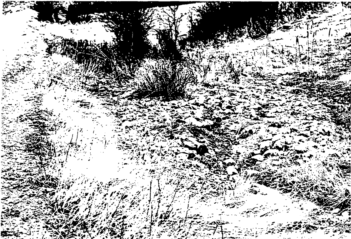
Photo 26: Cobbles transported by runoff from downpour and deposited along roadside.
