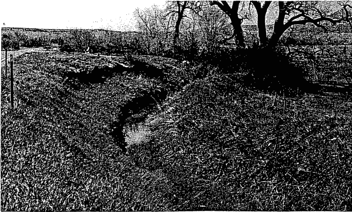
Photo 7. This is the section of Enterprise Ditch (Work Zone 5) that will be realigned; the old ditch section will be filled and revegetated. 4/18/01
