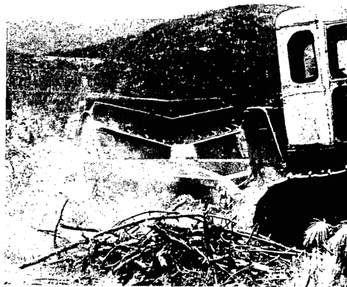
Huge piles of slash disappear in a flash, crushed by the roller chopper.
