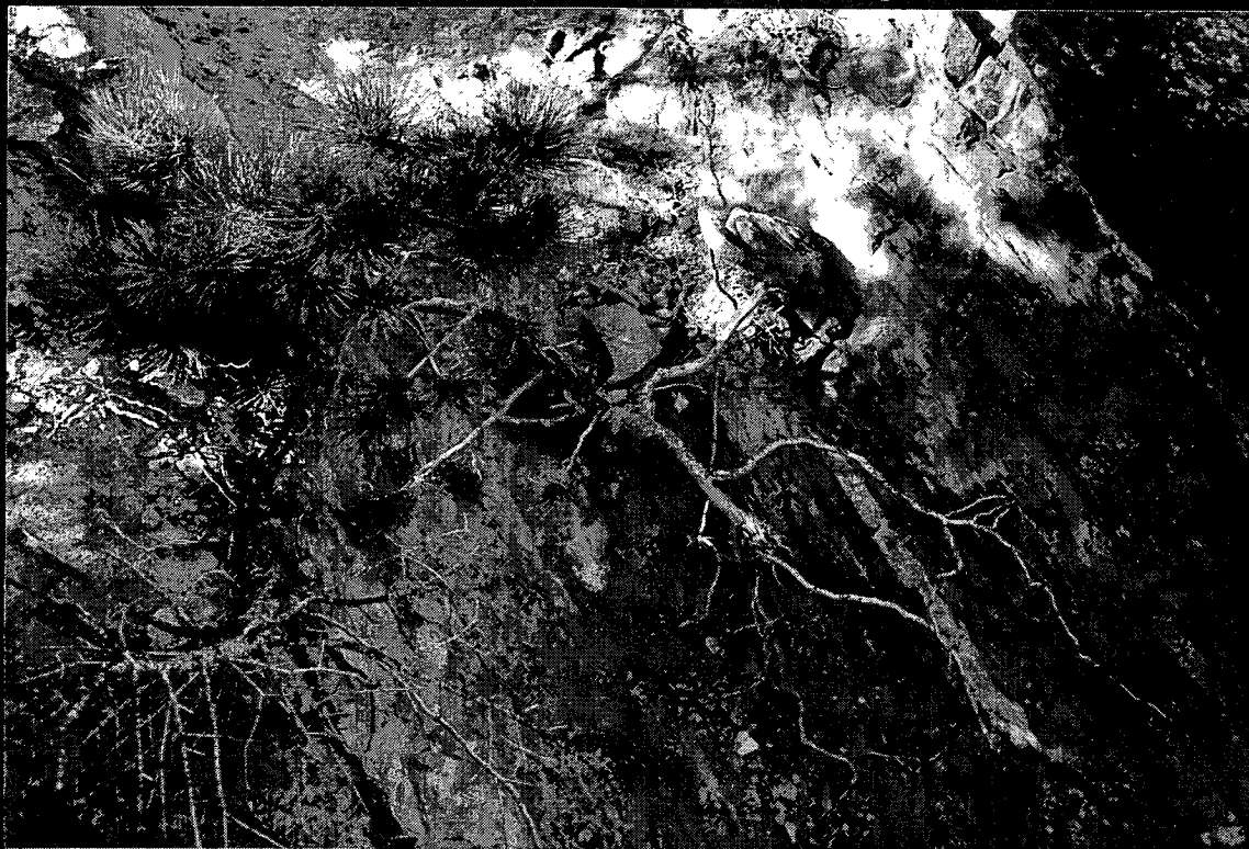
PHOTO #10: Exposed roots of a tree under Hueco Wall
