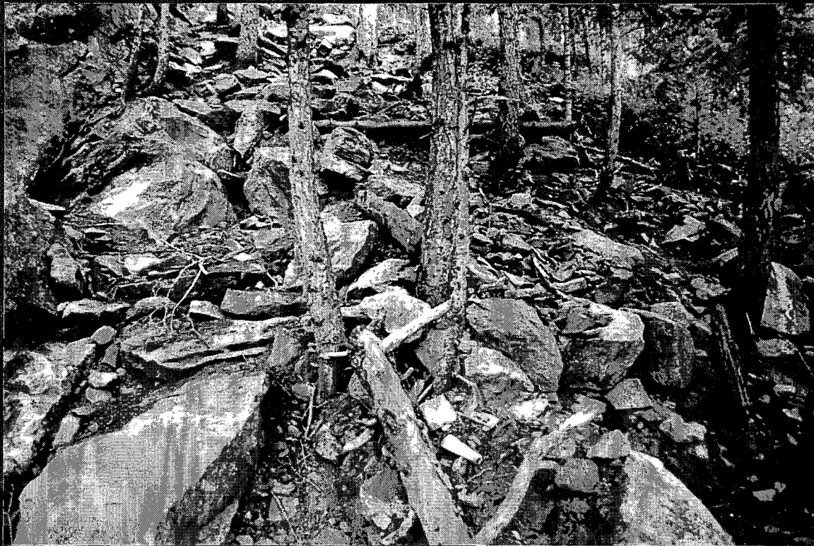
PHOTO #5: Eroded area on the north side of the Third Flatiron, near the top, looking west.
