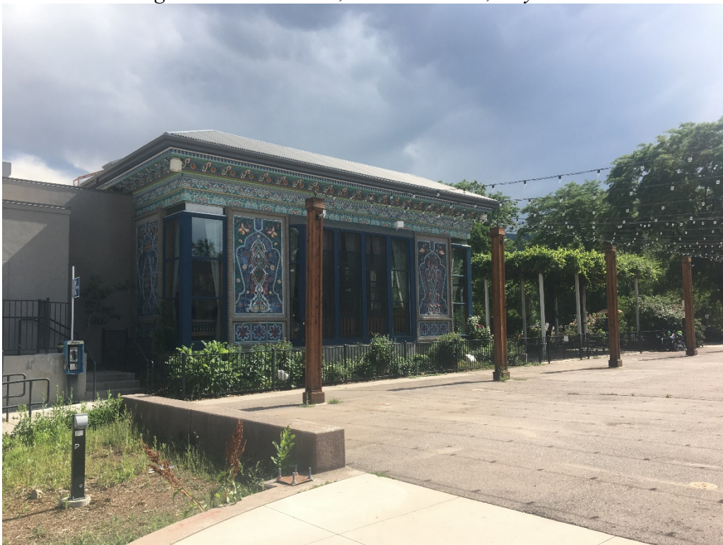
Figure 2. 1770 13 th St., North Elevation, July 2020.
