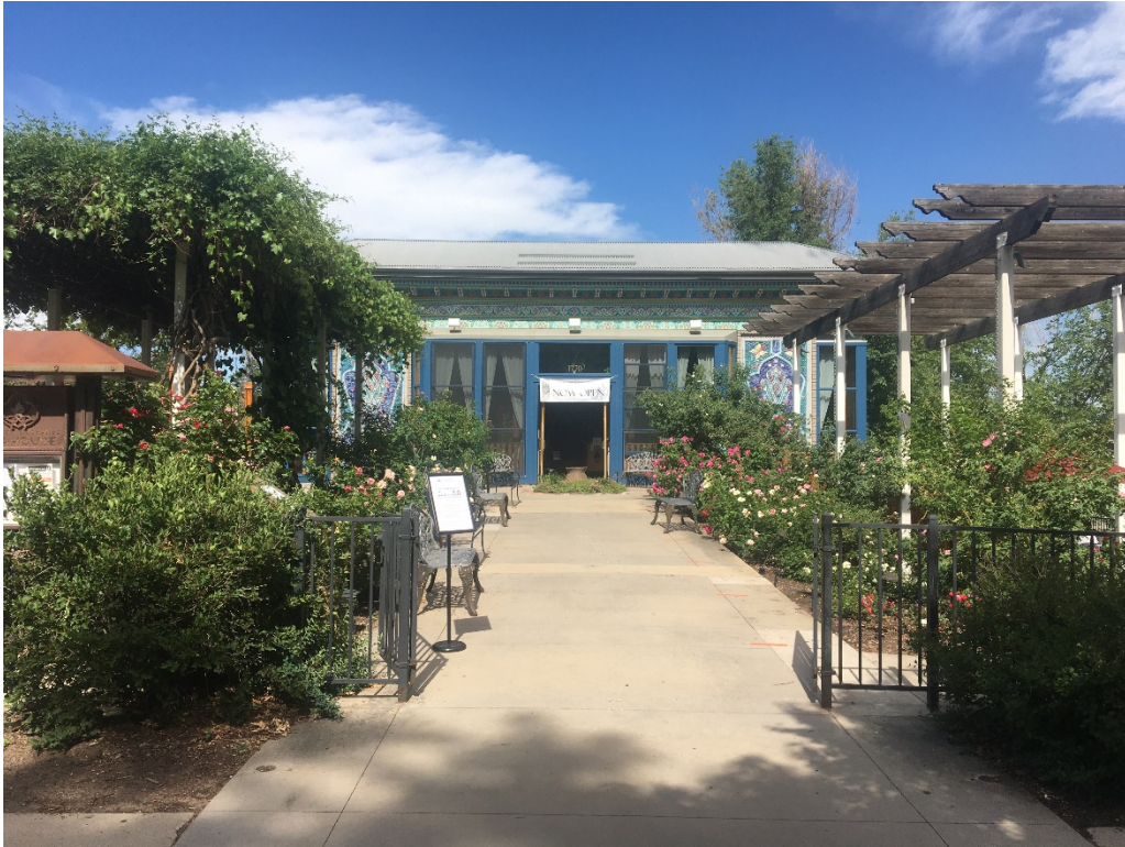
Figure 1. 1770 13 th St., West Elevation, July 2020.
